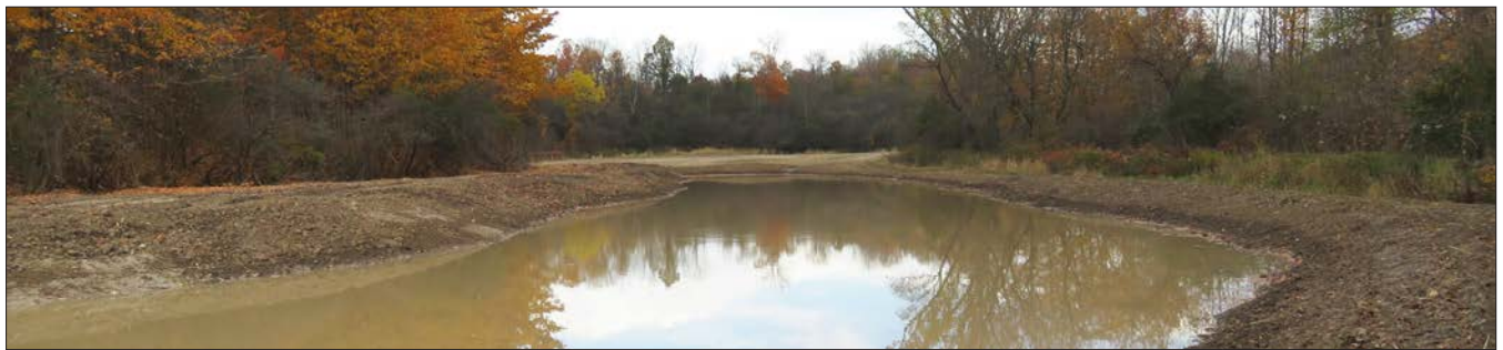
2022 – A 0.83-acre wetland restoration in Upper Parkhill watershed.
