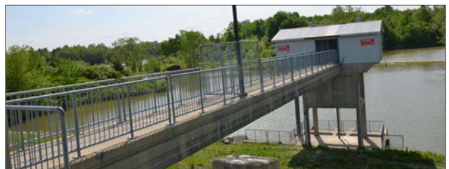
Parkhill Dam control structure.
