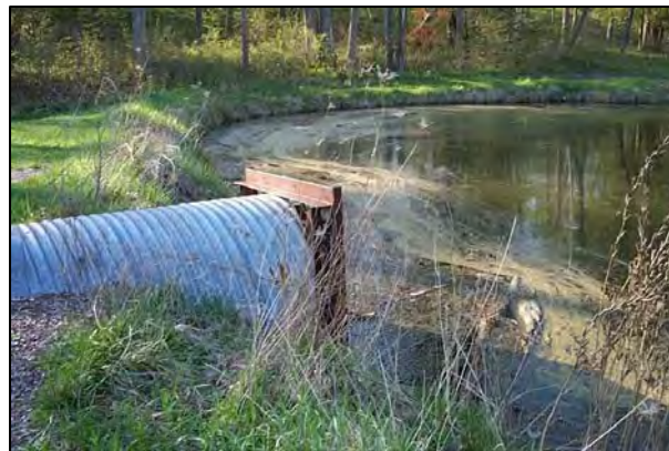
Pinedale Road Culvert
