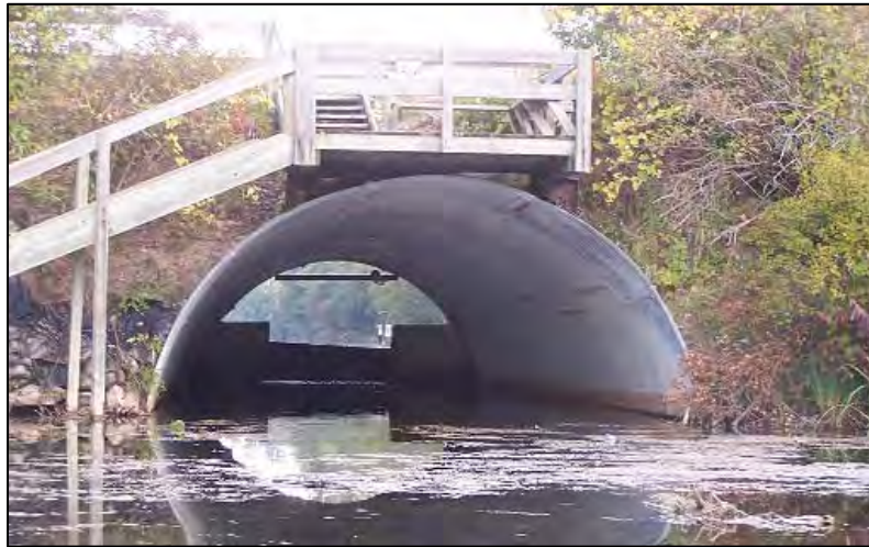
Pinery Park Dam, looking upstream through culvert at the bridge
