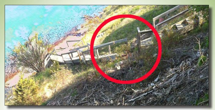
Slope instability indicators include displaced posts and fences, poles, monuments, guardrails, broken or displaced retaining walls, and stairs, among other indicators mentioned in this fact sheet. Please read the Recommended Management Practices panel inside.
