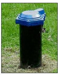
A properly-maintained wellhead can limit potential pathway for pollutants to reach groundwater sources.
