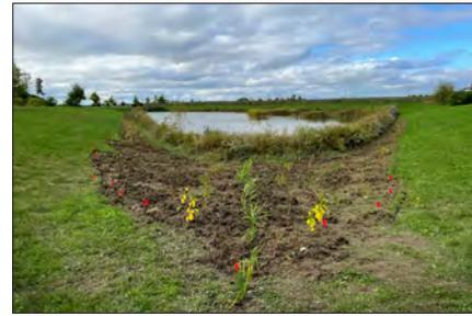
October planting at Campanale Stormwater Pond. This rain garden helps absorb nutrients and filter water runoff from the subdivision.
