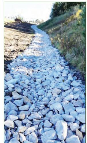
In photo at left, Parkhill Dam toe drain is shown prior to 2018 repair project. In photo at right, 2018 Parkhill Dam toe drain repair project is shown.
