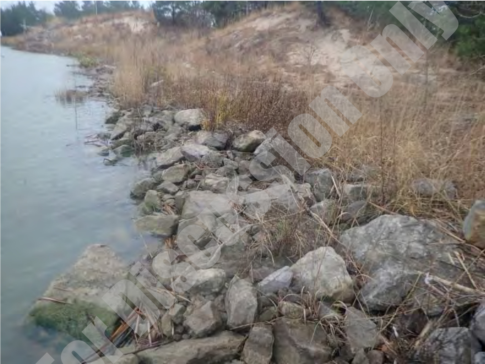
Photo B-17: North end of Reach 3, looking south.
