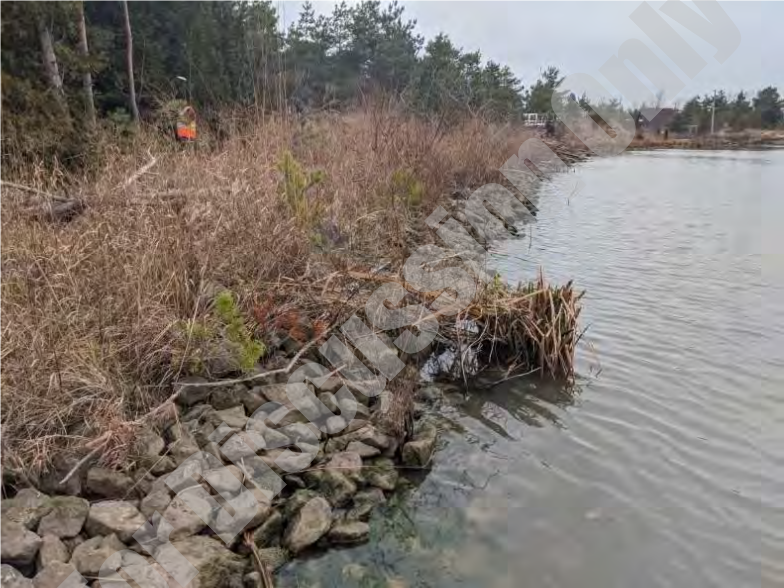
Photo B-2: Southern end of Reach 1, looking north.
