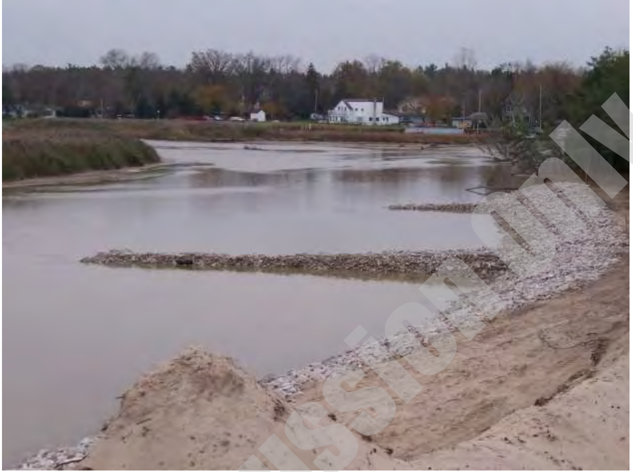
Photo A-1: Post-construction rock revetment and bend way weirs, looking south (taken 2006)
