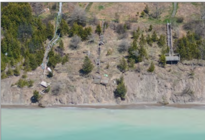
Slope instability causing failure of beach access stairs.
