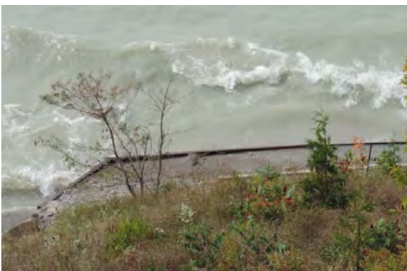
Steel Walls at base of steep slope
