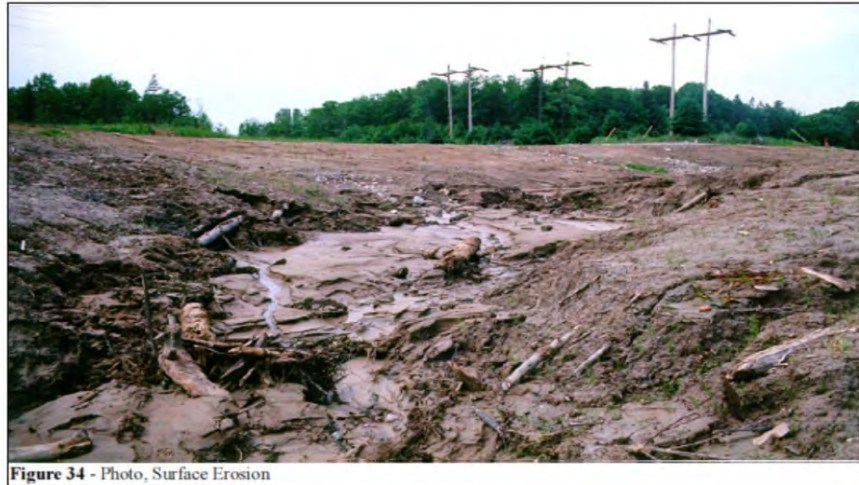
Figure 7.4: Surface Drainage Issues, From MNR – Figure 34, Terraprobe, Geotechnical Principles for Stable Slopes (1997) Page 37
