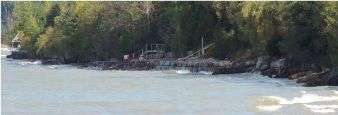
Ad-hoc, piecemeal shoreline protection works.
