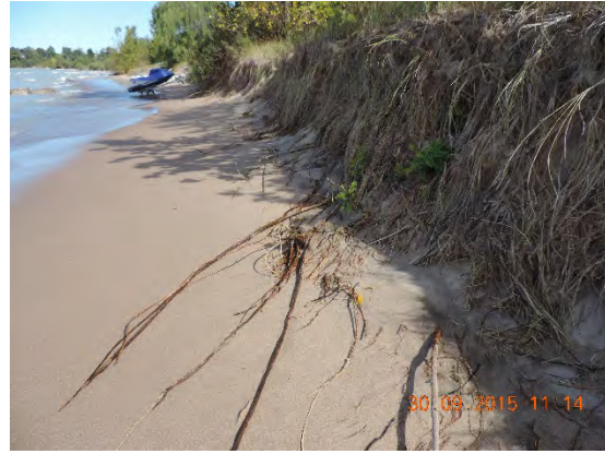
Grass systems being undermined and removed.
