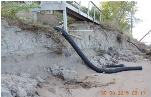
Undermining, breaking off and slumped materials along the eroding ABCA shoreline.
