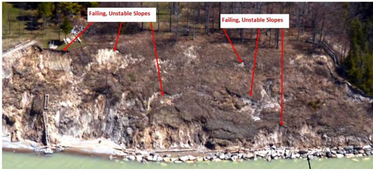
Protection Works along toe of slope
