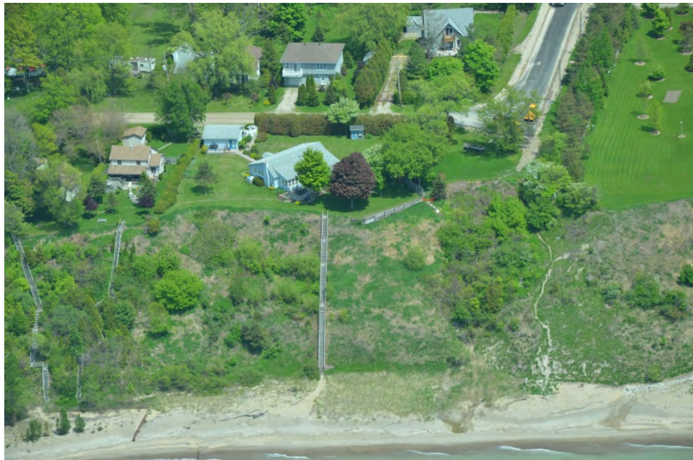
Figure 5.18: Oblique aerial photograph of a portion of the ABCA shoreline south of Bayfield showing a dynamic beach backed by an eroding cohesive bluff.
