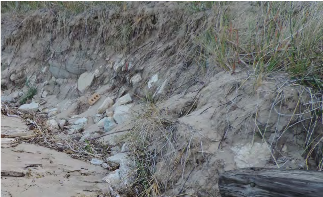
Poor quality materials (e.g. bricks, concrete rubble) of insufficient size remain from being washed out.
