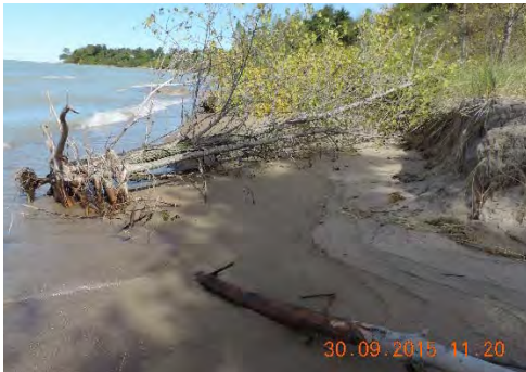
Erosion along shoreline (trees in water)
