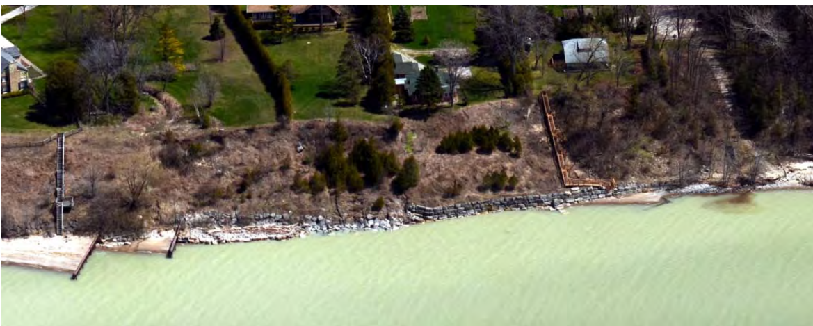
Ad-hoc, inconsistent, piecemeal shoreline protection works.
