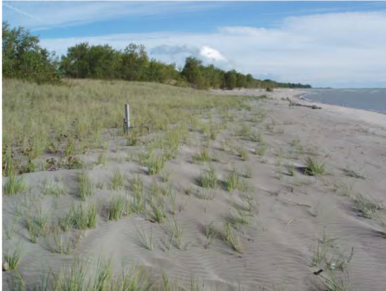
Figure 5.11 a & Figure 5.11 b): Erosion and recovery from a large storm, Long Point Provincial Park, Lake Erie: a) photograph taken after the storm of December 2, 1985 showing erosion of the foredune by 15-20 m. Note the tree stumps on the beach and the narrow, flat beach; b) the same site in 2008 showing a wider, higher beach and accretion of the foredune by wind completely burying the old dune scarp. Note that the lake level is considerably lower in 2008 than in 1985 thus permitting the foredune to build lakeward.
