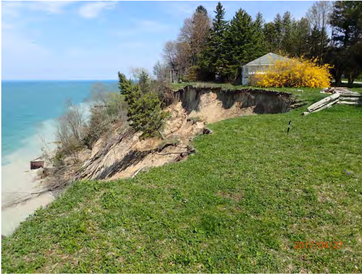
Figure 4.1: Residence located within the Erosion Hazard Limit on an actively eroding bluff on the ABCA shoreline
